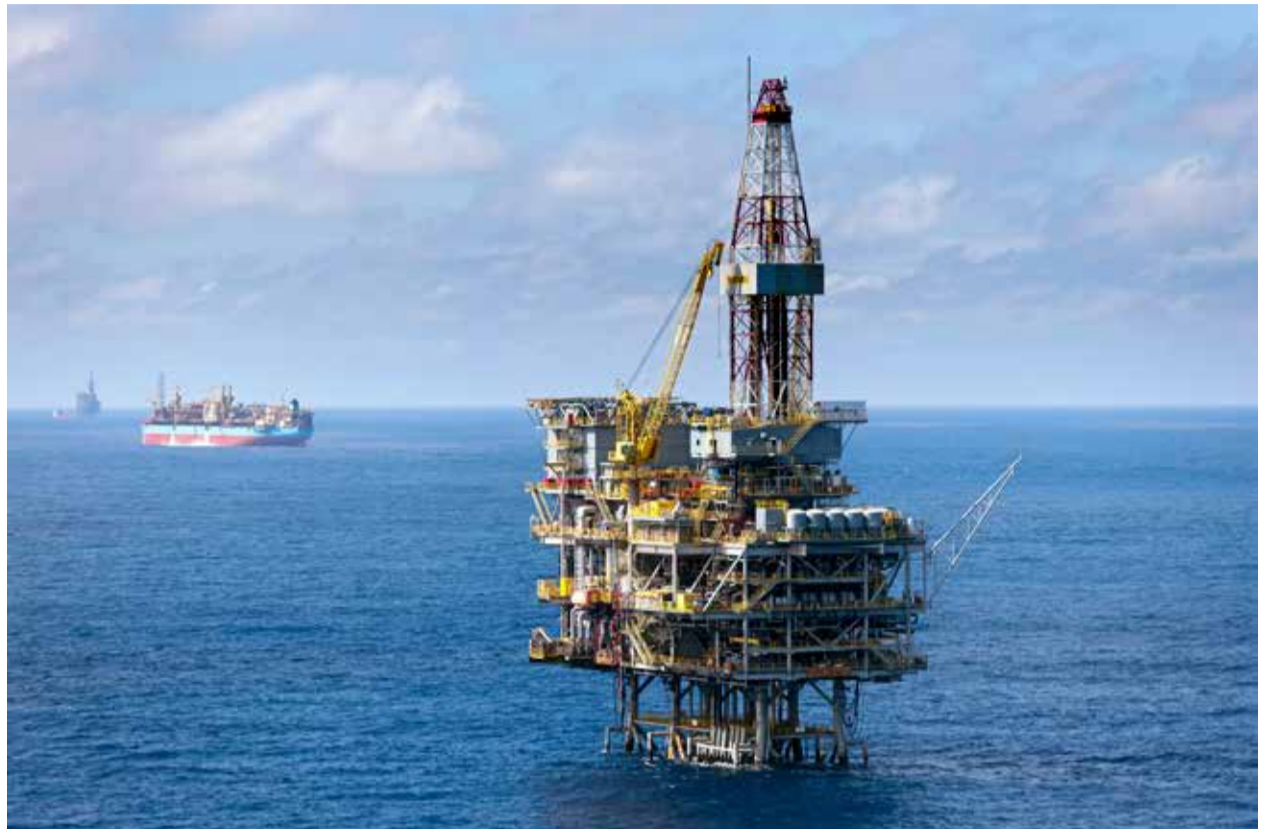
Ready for change: the Peregrino A platform with the Peregrino FPSO in the background
